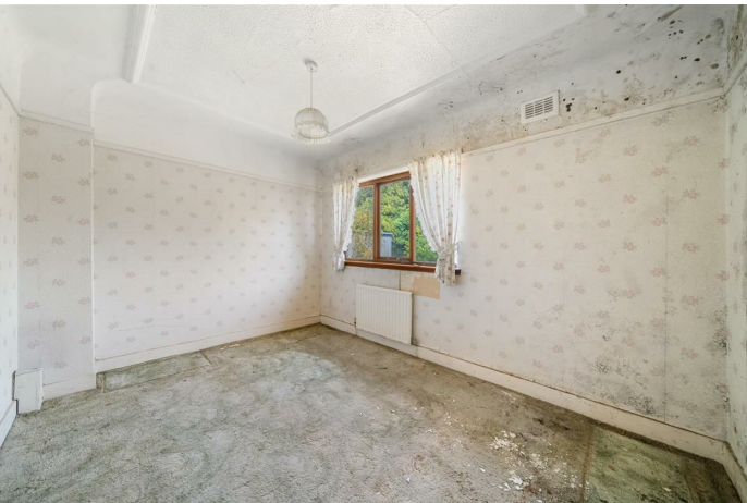
double glazed window to front aspect, radiator
